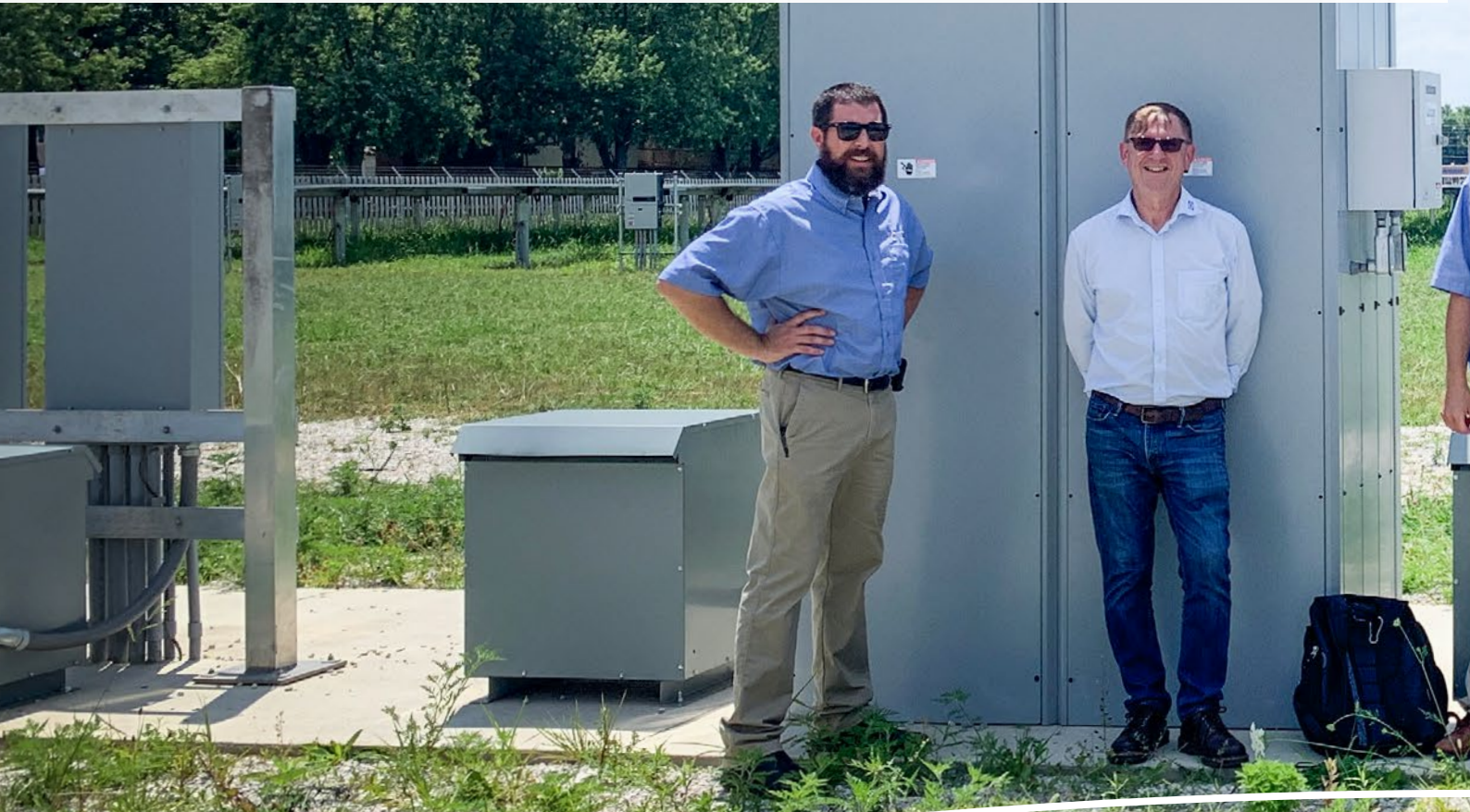
▲ The project team from left: Bob Cain (Director of Sales, Girtz), David Stringer (Business Development Manager, DEIF), Brent Beissler (Engineering Manager, Girtz), Greg Taylor (Sales Engineer), Jesus Davila (General Manager, DEIF) and Arash Habibi-Soureh (Distributed Energy Resources Manager, Johnson Melloh Solutions)
